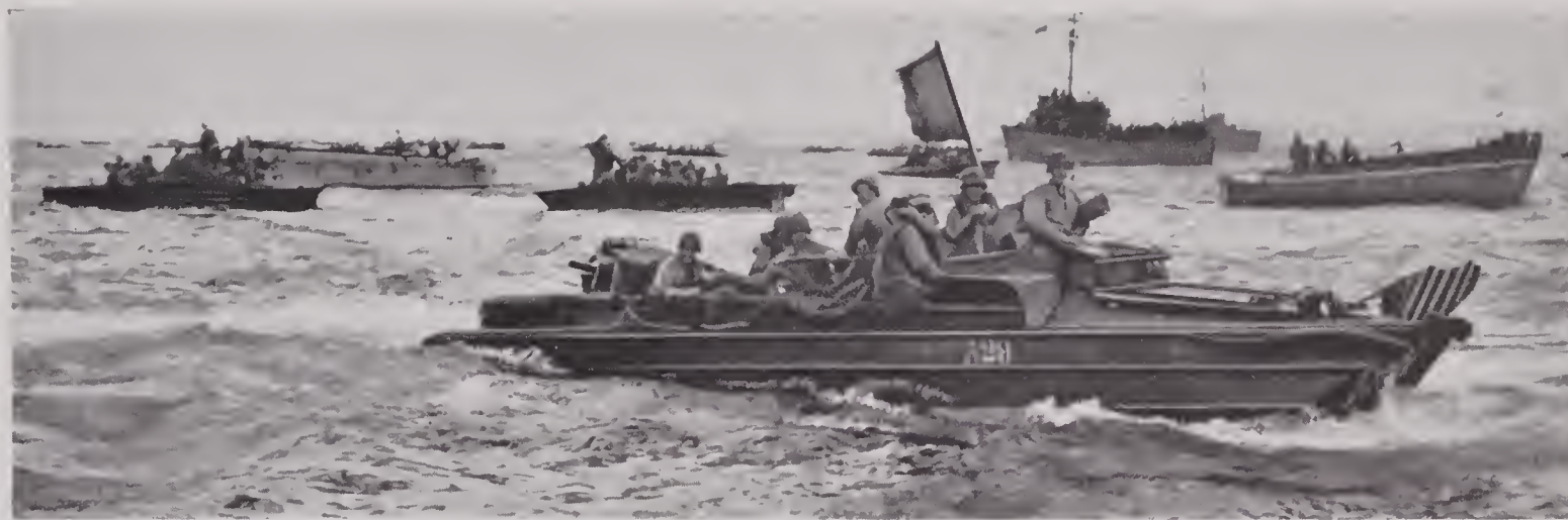
FIGURE 37. Marine Corps DUKW bringing in 105-mm howitzer during Guam landings.
